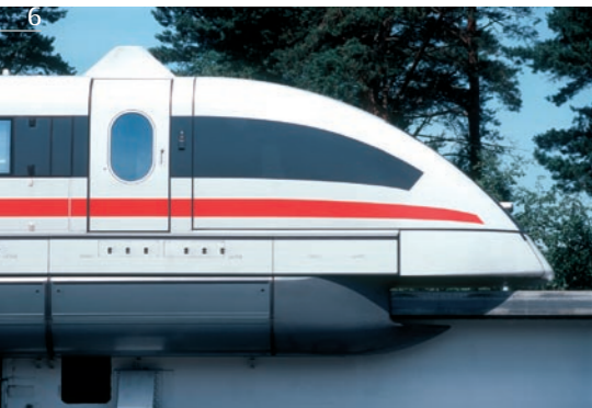
Transrapid unit on maglev guideway
